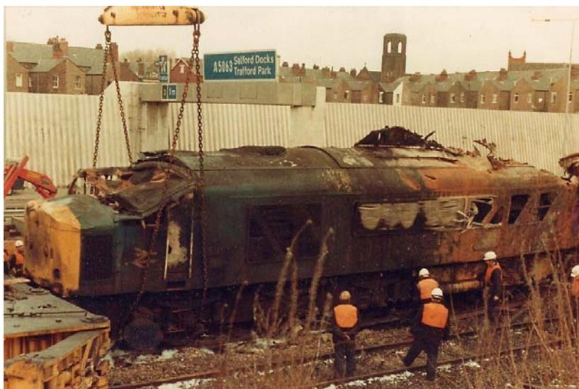
The front end (no.2 end) of 45147 was completely destroyed and the cab bulkhead driven almost horizontal into the engine compartment, although both
