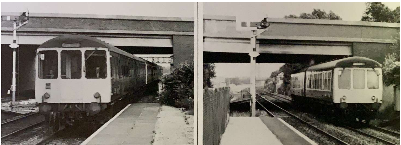
The semaphore Eccles ES50 signal pictured before the crash (left), showing the poor sighting against the bridge in the background, and after the crash (right) when it had been fitted with a white background. Eccles signal box can be seen beyond the bridge in the right hand picture.
