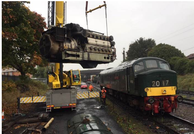
45125's repaired power unit is lifted back in at Loughborough on 19/10/17
