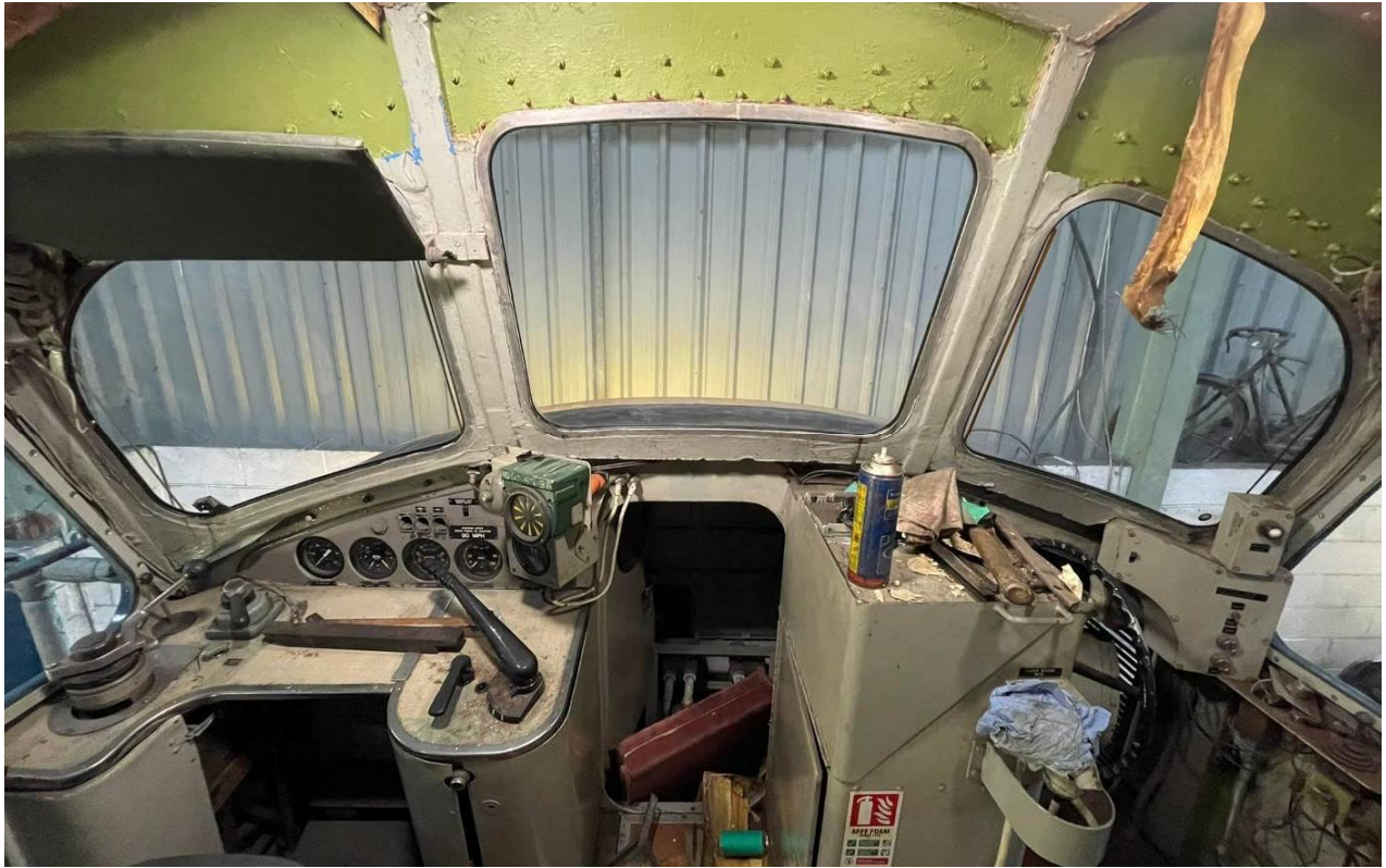
Two views of the cab windscreen glass reinstated at both end of 45133 by Pioneer Diesels Ltd. 20/05/22.
