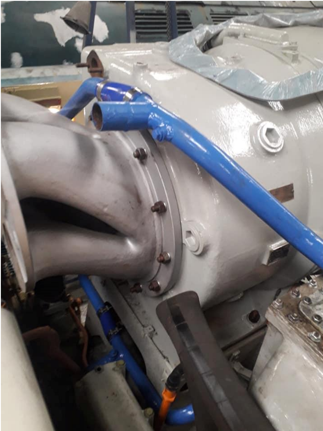
Coolant pipes (painted blue) being refitted to the turbocharger area. 24/07/22.
